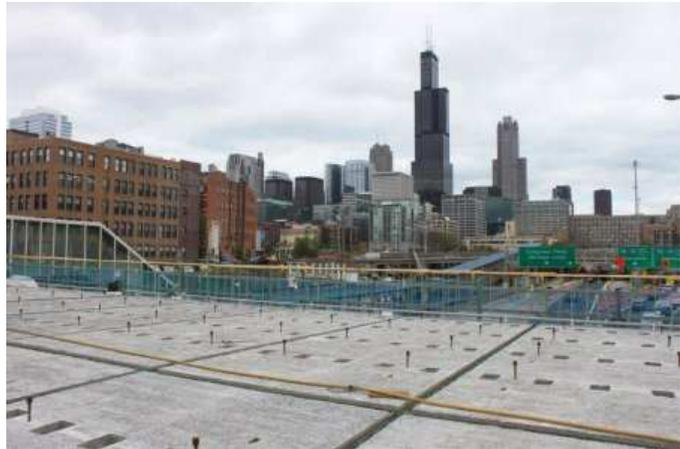
Precast deck panels, manufactured by Utility Concrete Products of Morris, were installed this summer on the new Peoria Street pedestrian bridge above Interstate 290 in Chicago
