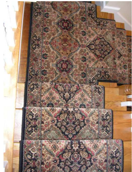
Submitted photo. A new installation technique shows a stairway runner pattern uninterrupted as it turns going down the stairs.
